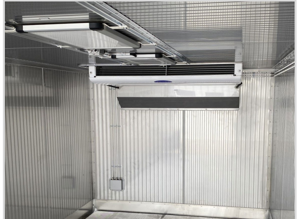
REFRIGERATOR UNIT INTEGRATED UPPER PART OF WALL
