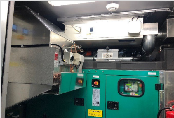
GENERATOR AND VENTILATION INTEGRATION
