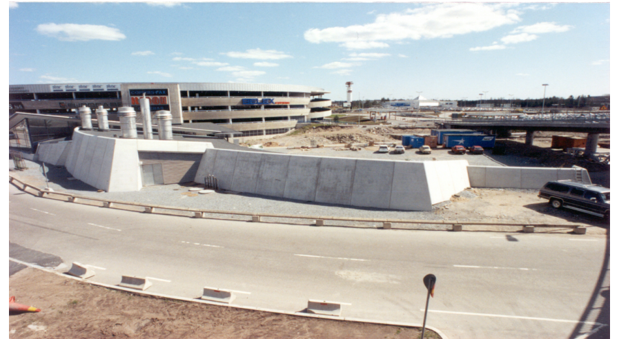
Reserve Power Station.
