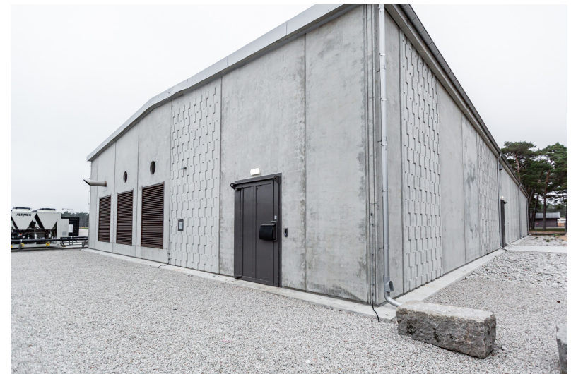
Grade VI protected infrastructure (generators, chillers etc).
