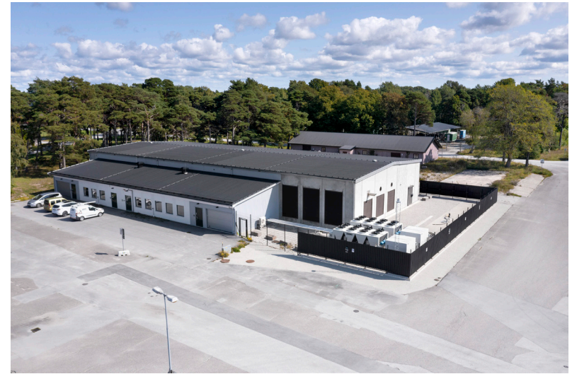
Grade VI high security data center.
